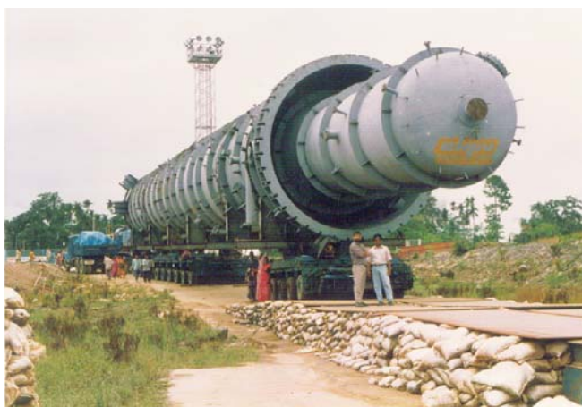
Atmospheric column being brought from Jetty.
