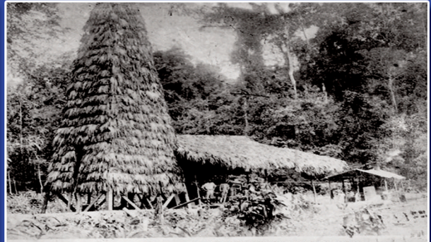
DRILLING WELL COVERED BY THATCH IN DIGBOI, 1905
