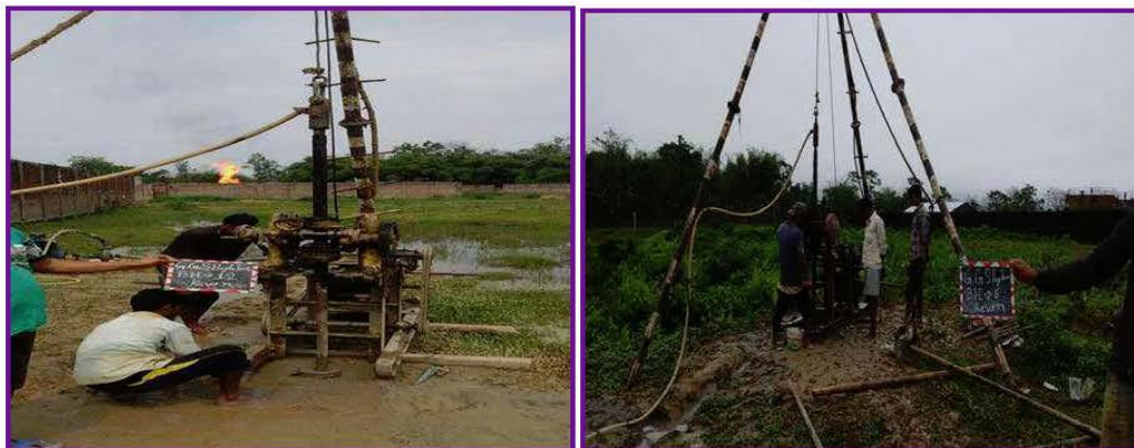
Fig. 3: Soil Exploration in progress at location BH-12 & BH-6 for the Proposed Group Gathering Station (GGS) at Baghjan, Tinsukia Assam
