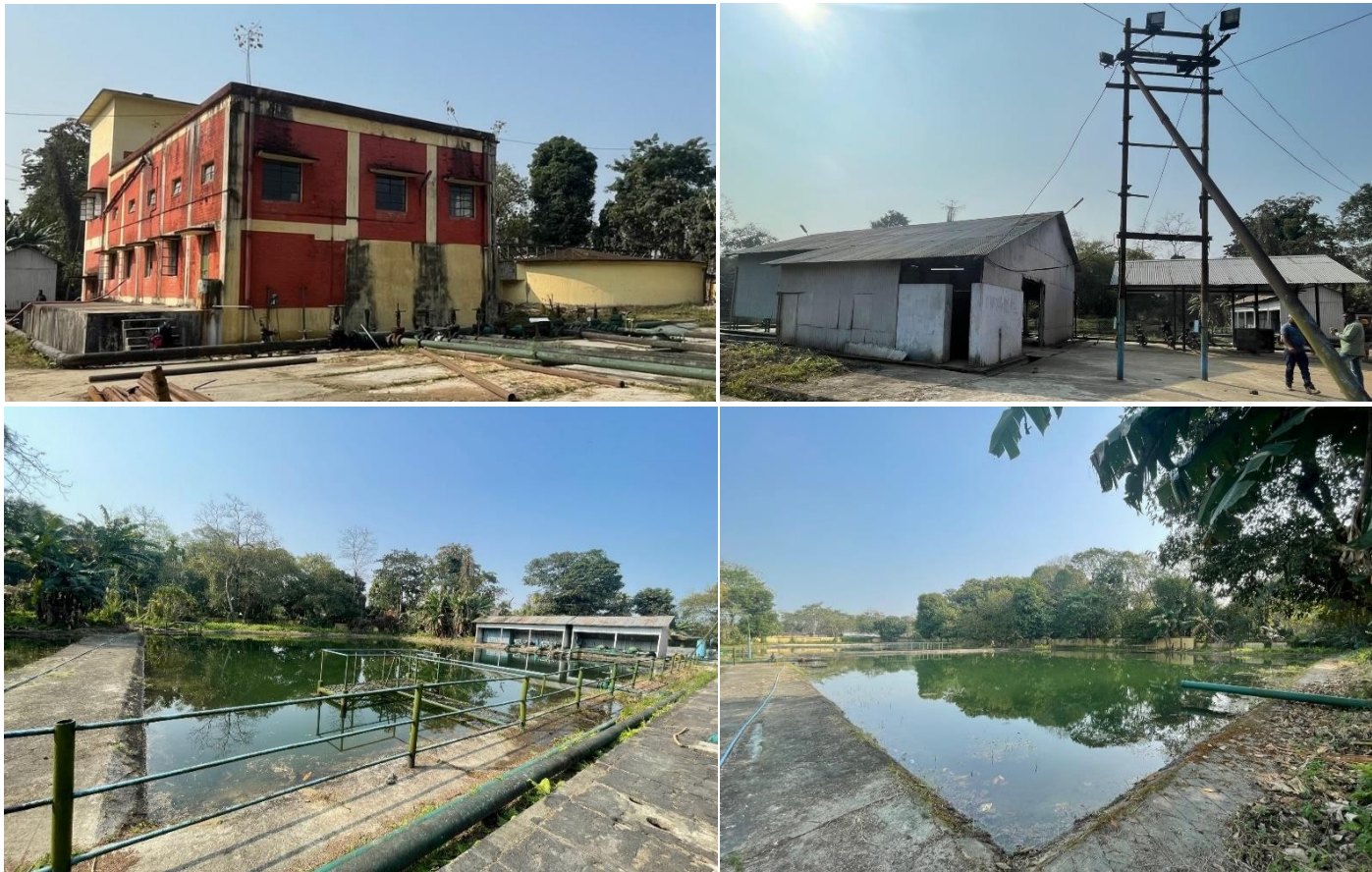
Fig: Indicative Photographs of old 1.5 MGD WTP
